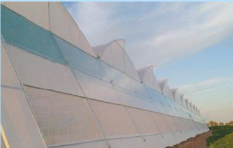
NVPH HEVY STRUCTURE
