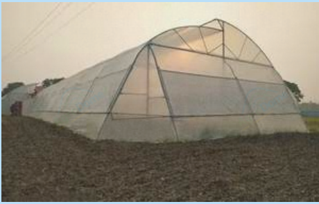
SINGLE SPAN NVPH
