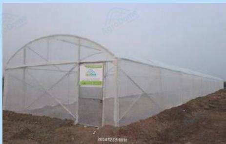
SINGLE SPAN TUNNEL
