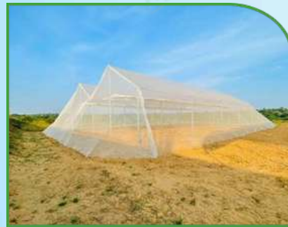
Wire Rope Polyhouse
