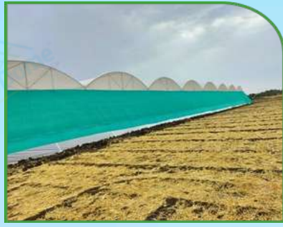
Dome Roof Net House -DRNH
