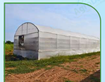
Solar Dryer Structure
