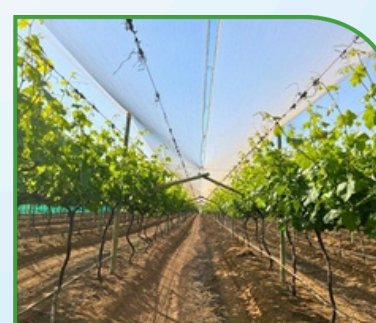
Grapes Orchard Sliding Structure
