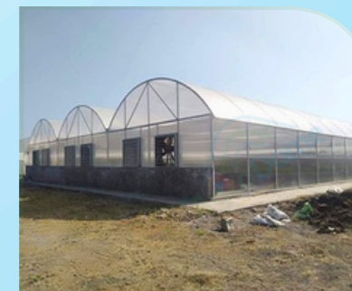
Poly Carbonate Structure
